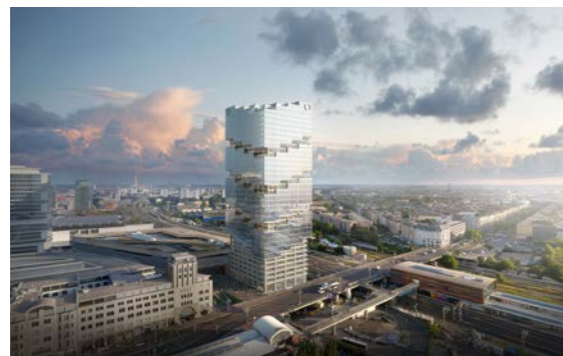
EDGE East Side Berlin, Berlin, Germany A joint venture with German pension fund BVK, this forward purchase of a development in Berlin’s Mediaspree sub-market will, once complete, be one of the most hi-tech, sustainable office buildings in Europe.
