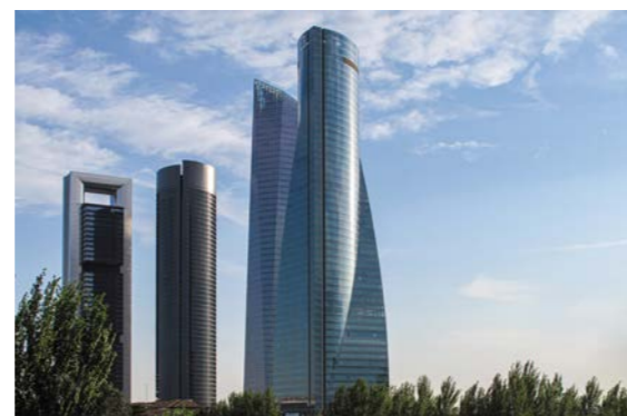
Torre Caleido, Madrid, Spain Allianz provided a 10-year loan alongside Caixabank to fund the development of a mixed-use office and retail asset to stand alongside the four existing towers in Madrid’s Cuatro Torres Business Area.
