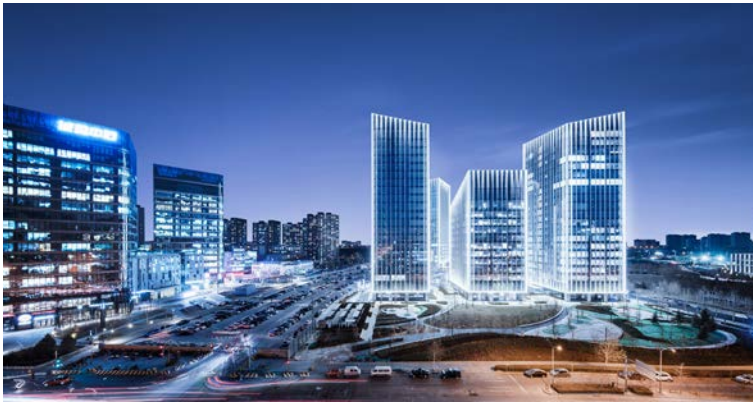
Ronsin Technology Center, Beijing
